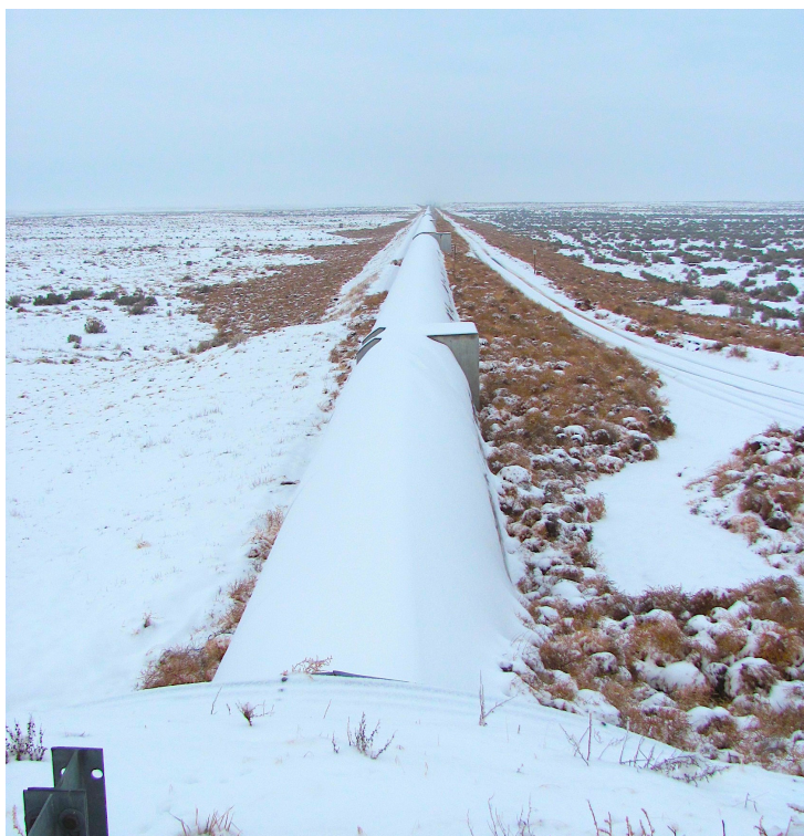
9-1 One of the 4 km beam tubes at LIGO Hanford. A strange alien structure in the middle of nowhere.
